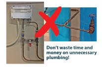
Remote sensors eliminate need for bypasses
