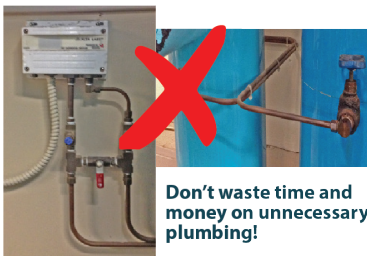
Remote sensors eliminate need for bypasses
